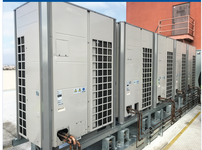
FIGURE 2 VRF heating and cooling system.
